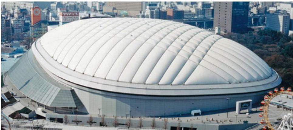
Figure 1.3: Inflatable Roof of a Stadium in Tokyo, [8].
