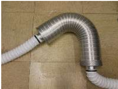
(c) Sound Attenuator (Silencer)
