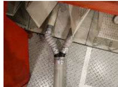
(e) Airflow Inlet to the Anechoic Chamber
